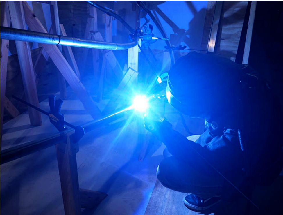
David Schurman tries his hand at some welding during the fabrication process.
